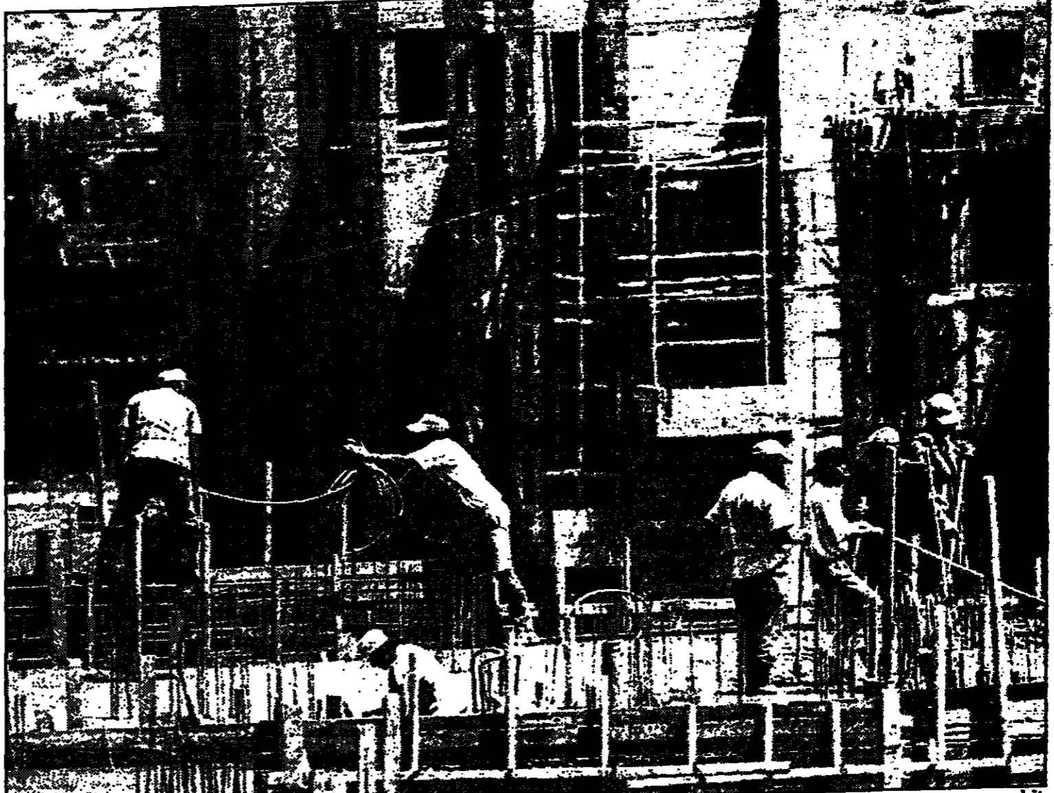
Palestinian workers pour concrete on the roof of an apartment building in Kiryat Sefer yesterday. The government announced it had lifted a construction freeze in the haredi settlement and plans to build another 1,806 homes there. (Razzer)
